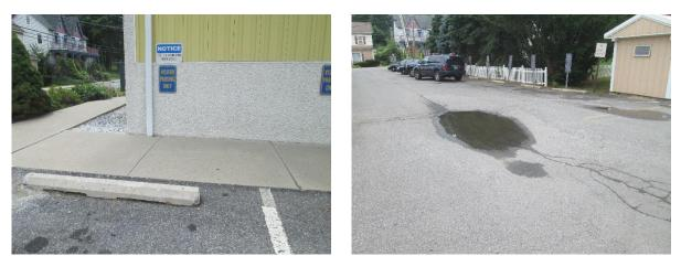
Parking spots to the north of the building can be replaced with porous asphalt to capture and infiltrate stormwater. Runoff from the roof top can be disconnected and drain into the rainwater harvesting system. A preliminary soil assessment suggests that the soils have suitable drainage characteristics for green infrastructure.
