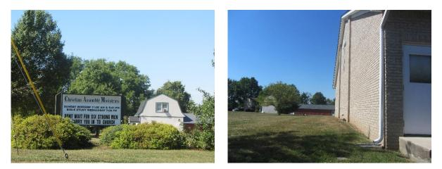
Parking spots in front of the building can be replaced with porous asphalt to capture and infiltrate stormwater. Installing a rain garden adjacent to the building can capture, treat, and infiltrate roof runoff. A preliminary soil assessment suggests that the soils have suitable drainage characteristics for green infrastructure.
